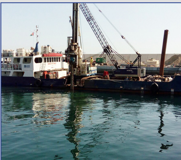
Pre-drilling rock for pile installation
