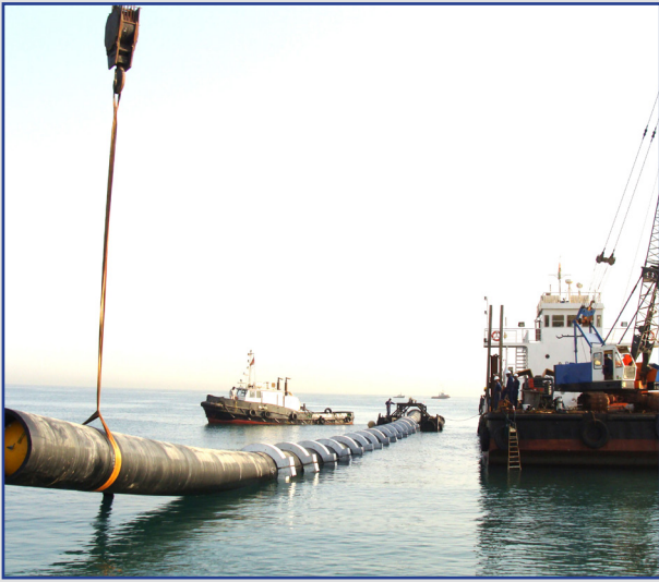
Installation of HDPE pipeline
