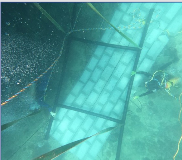
Divers installing concrete mattress
