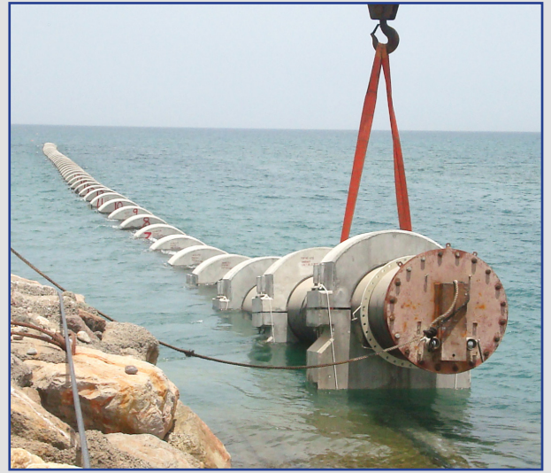
Launching 1800mm HDPE pipe
